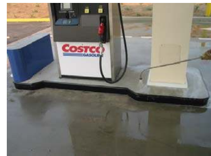
A simple spray application of CMW
